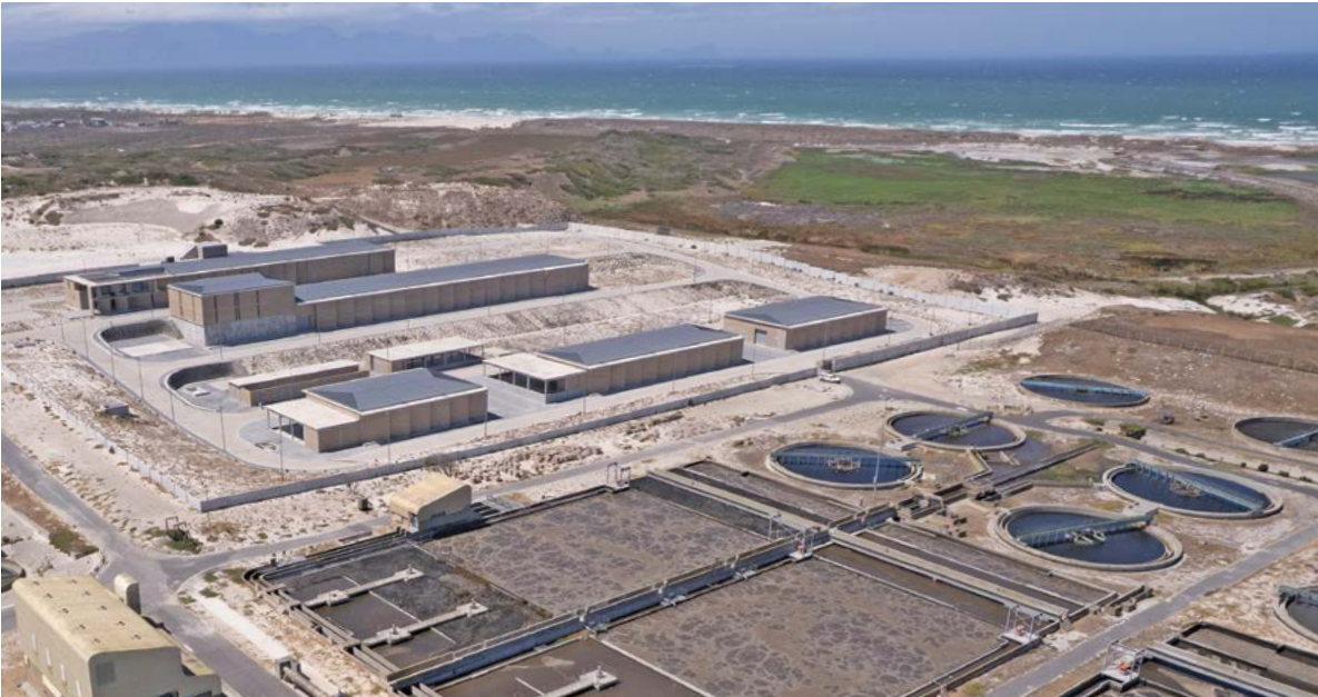
Getting there: An aerial view of progress with the Cape Flats advanced water reclamation plant, which is a vital part of the City's groundwater action plan to secure alternative water sources for Cape Town.
